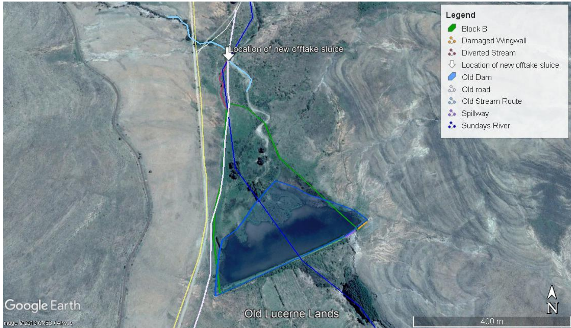
Figure 3: Block B prior to the development
