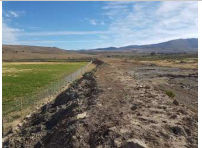
Figure 4: The diversion channel for the Sundays river with the lowest dam bay of Block A to the left
