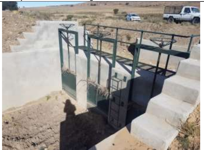
Figure 10: The big off-take sluice gate, photographed from the East
