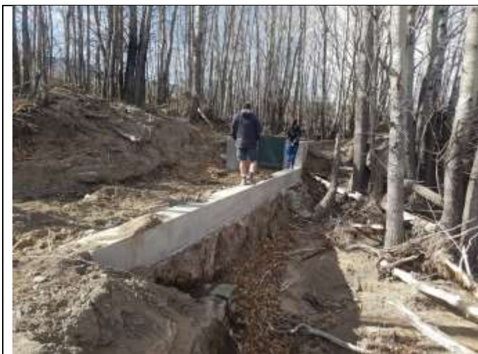
Figure 13: The off-take sluice and weir that diverts water to the feeder canal towards Block A
