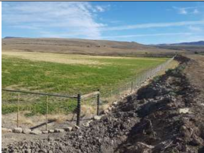
Figure 3: The lowest dam bay of Block A with the berm of the diversion channel to the right
