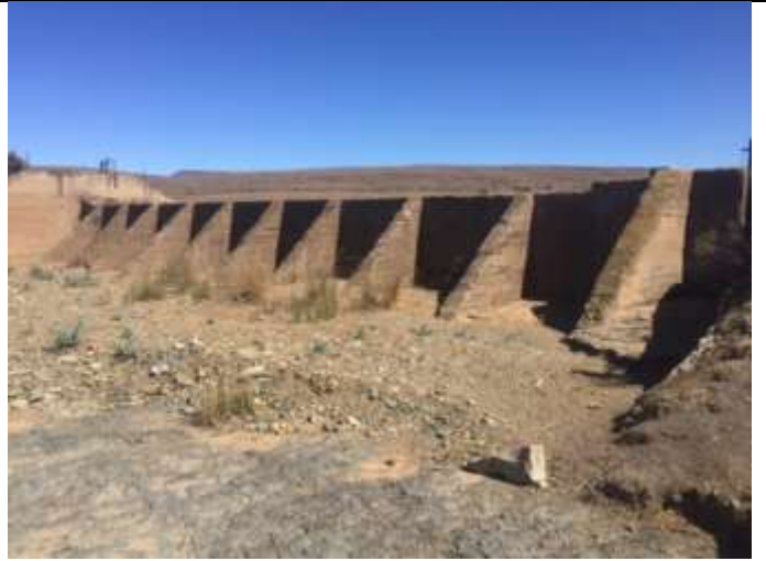
Figure 2: Spill way of the old dam
