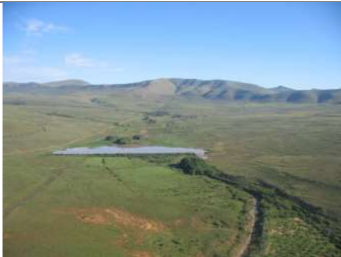
Figure 21: The old dam before the development took place, with the old fallow lands visible in the foreground in the right hand corner
