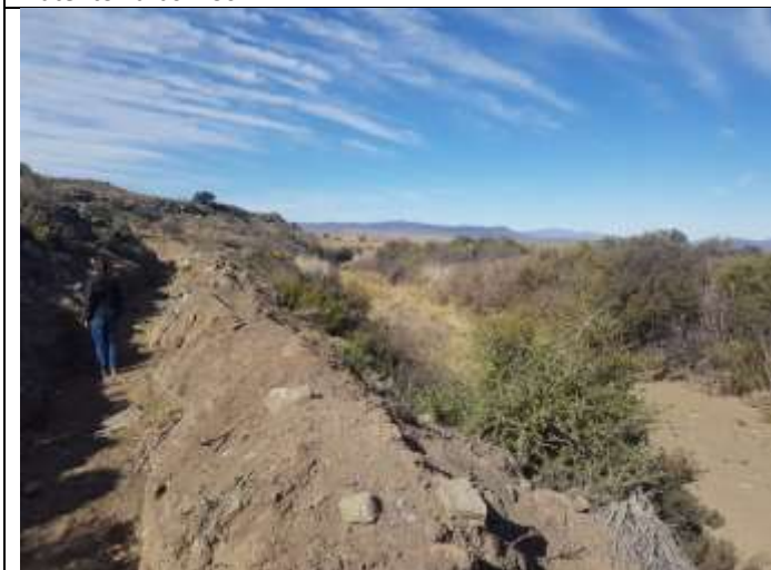
Figure 17: The feeder canal that diverts water towards Block A and the dry Sundays River
