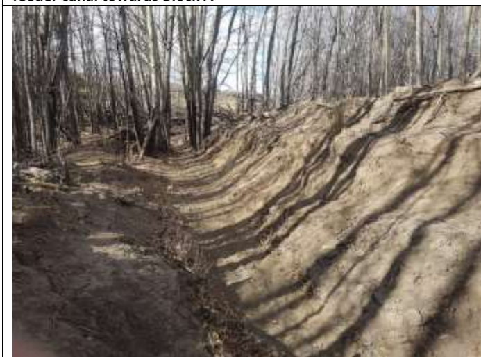
Figure 15: The feeder canal behind the off-take sluice that diverts water towards Block A
