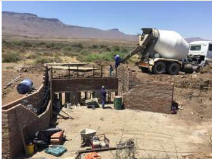
Figure 23: The construction of the big off-take sluice north of Block B
