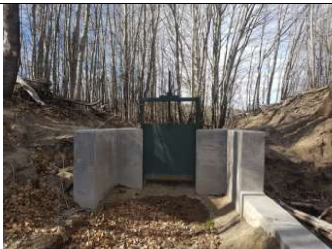
Figure 14: The off-take sluice that diverts water towards Block A
