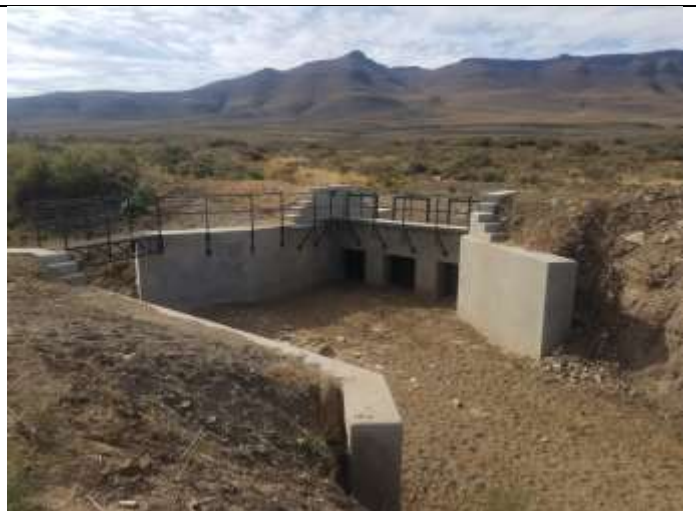
Figure 12: The big off-take sluice gate situated north of Block B
