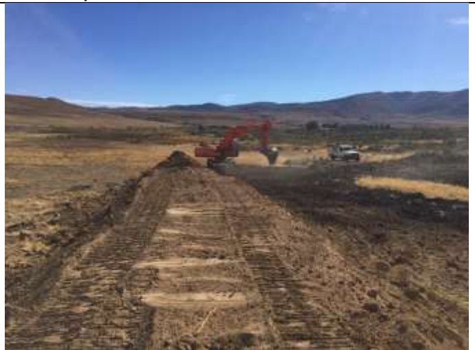
Figure 22: the construction of the diversion berm next to Block B
