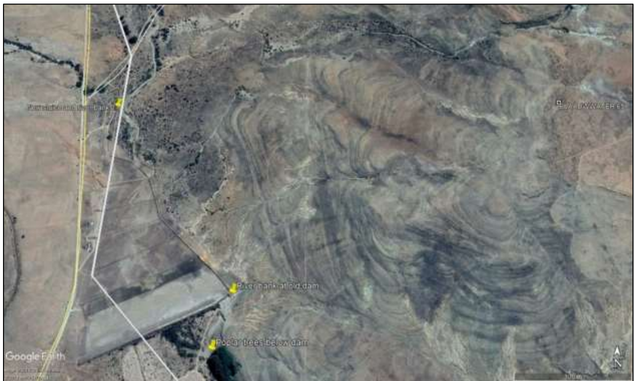
Figure 1. Google Earth aerial image showing the location of the newly-constructed sluice gate, 'upstream' to the north-west, diverting floodwaters to the old dam. An old sluice gate and irrigation channel are located amid Poplar trees to the south-east, 'downstream' of the spillway of the old dam (which also feeds a series of flood-irrigation basins planted up with lucerne).
