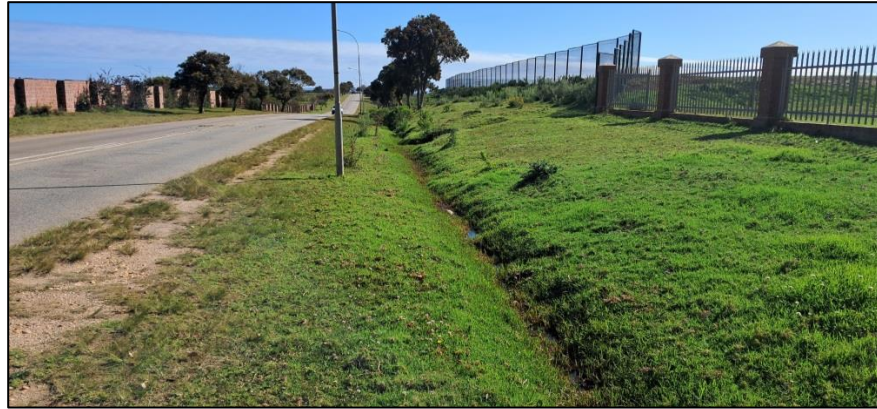
South westerly view:
