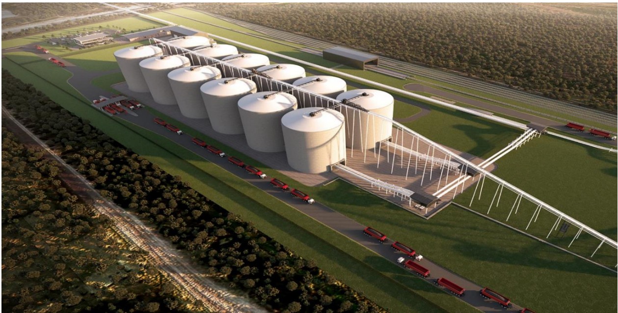
Figure 2-4: Illustrative example of the silos in and conveyor belt
