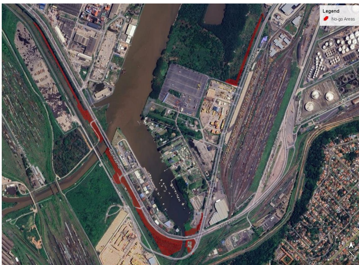
Figure 7-1: Areas to be avoided during construction (Edwards et al. , 2025).
