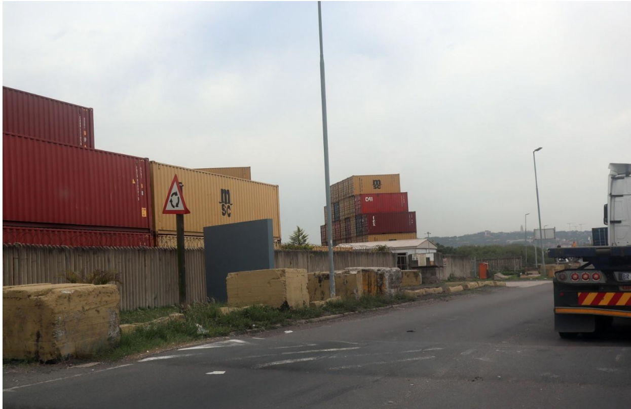
Figure 4, Plate indicating Traffic Management using Concrete Blocks on Bayhead Road
