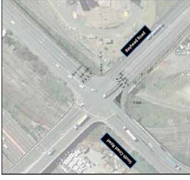
Figure 39 Bayhead / South Coast Road Intersection (TNPA, 2015)
