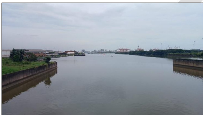
Photo 17: View of channel of Unit C02 looking from Bayhead Road downstream into the Durban Harbour.
