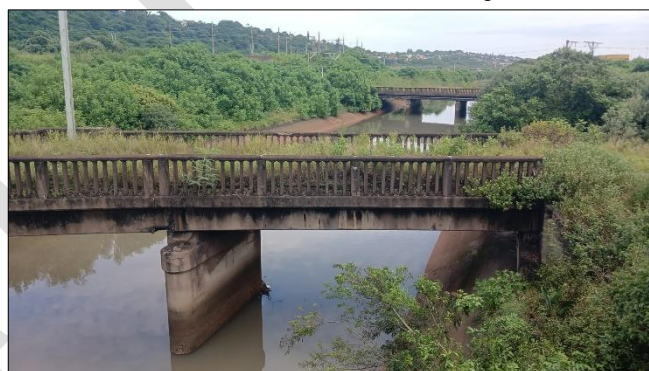
Photo 14: View of channel of Unit C01 looking upstream.
