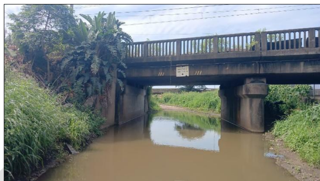
Photo 16: View of channel of Unit C02 looking downstream towards one of the bridges along Bayhead Road to the north.
