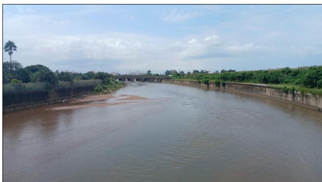
Photo 15: View of channel of Unit C02 looking downstream towards Bypass Road in the distance to the north.
