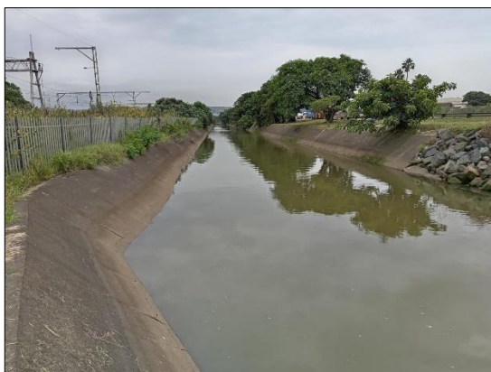
Photo 18: View of channel of Unit C03 looking upstream.
