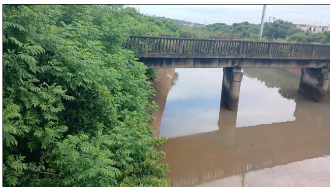
Photo 11: View of channel of Unit C01 looking upstream.
