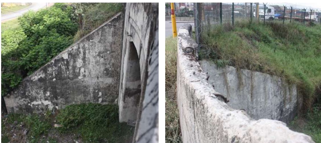
Figs. 14+15. Views of railway tunnel to Bridge B/2/5, 2026.
