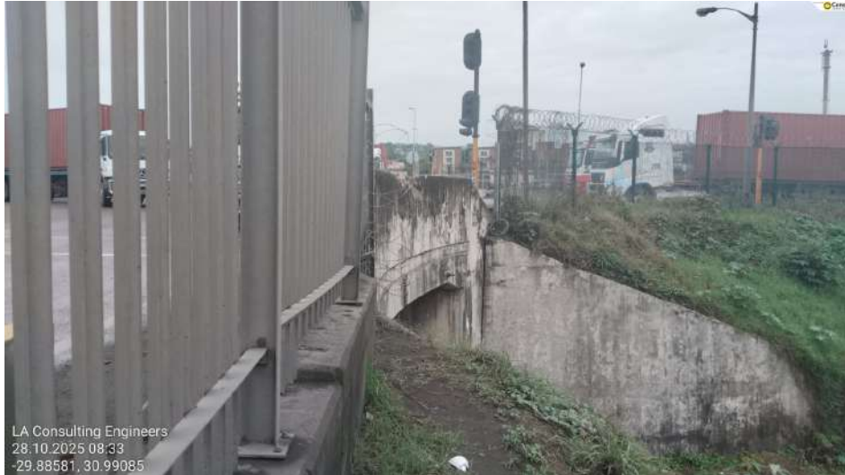
Fig.1. Street View: Bayhead Rd / South Coast Rd intersection. Oblique view from North-east of railway tunnel to Maydon Wharf, Durban, 2026.
