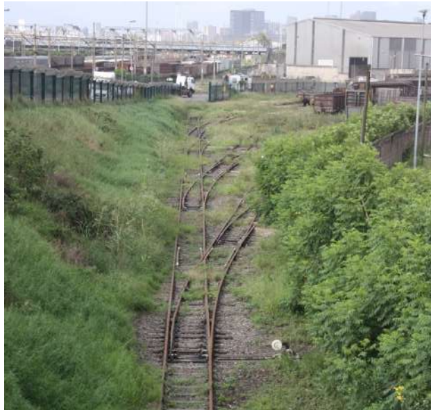
Fig.10. Maydon Wharf branch line, 2026.
